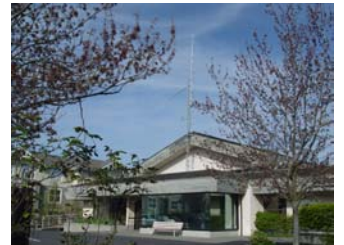
Red Cross House with ECT Antenna
